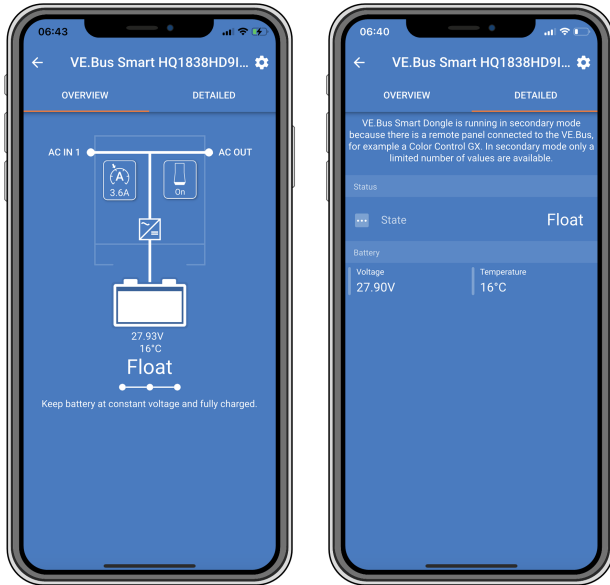
VictronConnect screens when the dongle is connected to a GX device.
